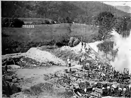
FIG. 5.—BRUSH AND STONE COFFERDAM, BULL'S BRIDGE.
